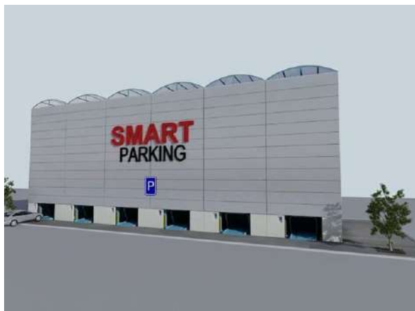
Figura 154: Exemplu de parcare smart parking (sursa: http://smartparking.ro/products/seria-l/# )
